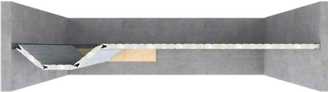
Wedge a single panel in between the two already placed panels. Make sure that the male and female connection points of the panel are positioned correctly.
