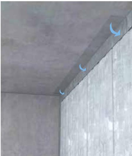
Once all K8 SUPAPANEL® are slotted into the track, fold the flange against the wall.
