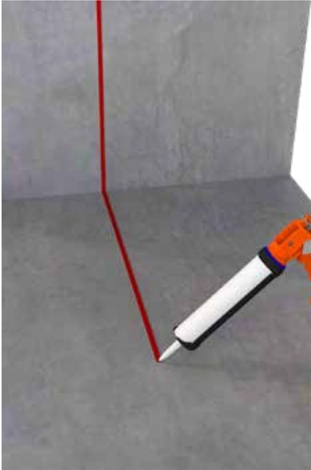
Before track is fixed to the structure, place a continuous bead of sealant on the surface where the track will be installed.
