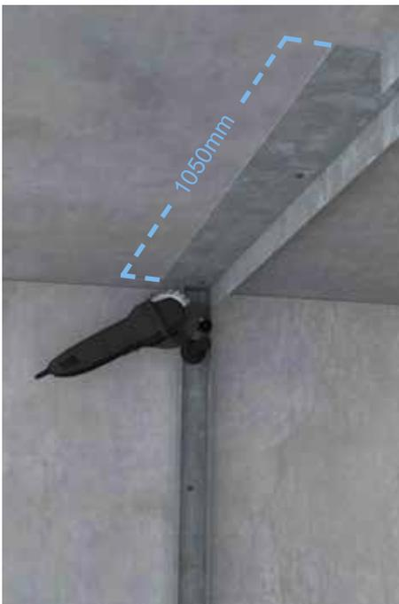
It is highly recommended to cut a flange at 1050mm wide into the top track as this will help slot K8 SUPAPANEL® into the track and close off the wall.
