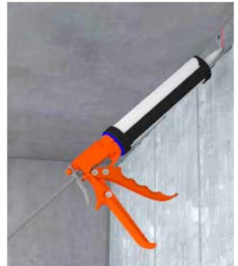
Place a bead of sealant within gaps to seal the flange.
