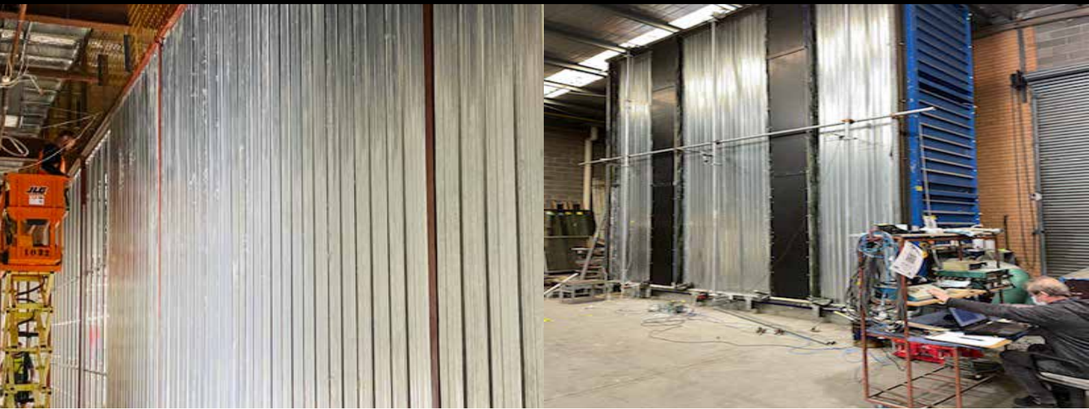
K8 SUPAPANEL® wind test being performed
