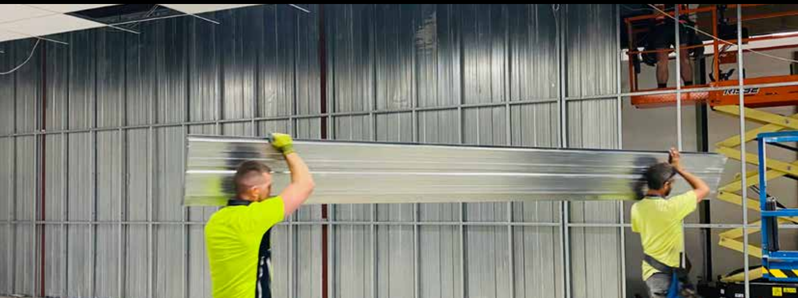
K8 SUPAPANEL® onsite install
